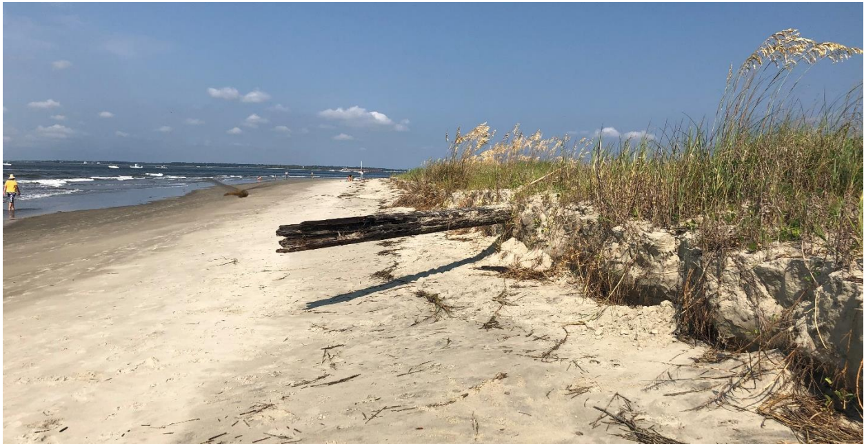
Figure 14. Area of significant shoreline change (erosion) in Figure 12. The buried engineered pile (probably a relic of an earlier storm) is extended seaward about 10 feet and 2-3 feet above active beach profile.
